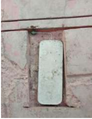
(a) Type – I (Conventional galvanic anode)
