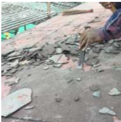
(a) The micro-concrete top overlay was removed by chipping by hand
