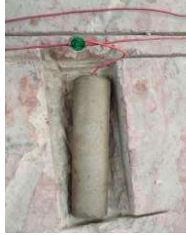
(b) Type – II: (Two-stage hybrid galvanic anodes)
