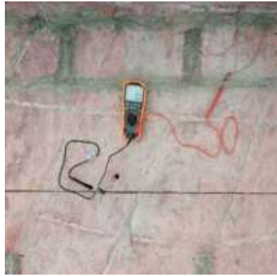
(e) Electrical connectivity was checked using a multimeter
