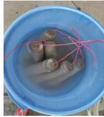
(f) Anodes were pre-wetted to saturate the encasing mortar
