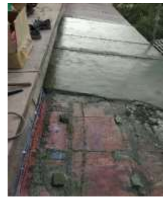
(i) Weathershade was covered with 20 mm thick waterproofing overlay
