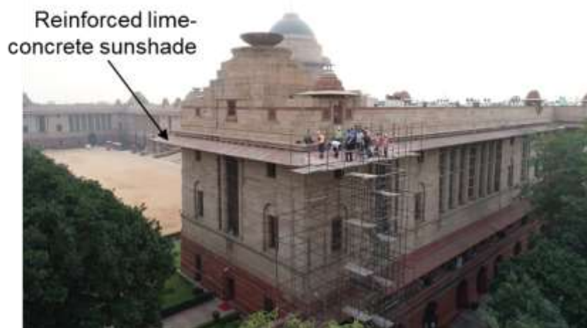
Figure 4.3: Pilot Project site at the heritage structure in New Delhi (Photo courtesy: CPWD, Rashtrapati Bhavan)
