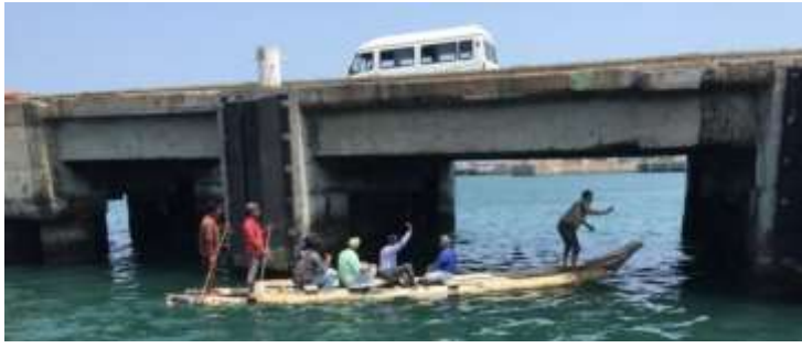
(a) Repaired piers of finger jetty (Photograph taken in 2019)
