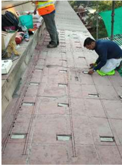
Figure 4.10: Installation of galvanic anodes in saw-cut pockets on the weather shade
