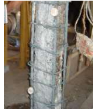
(c) Anti-corrosive chemical coated on the concrete surface
